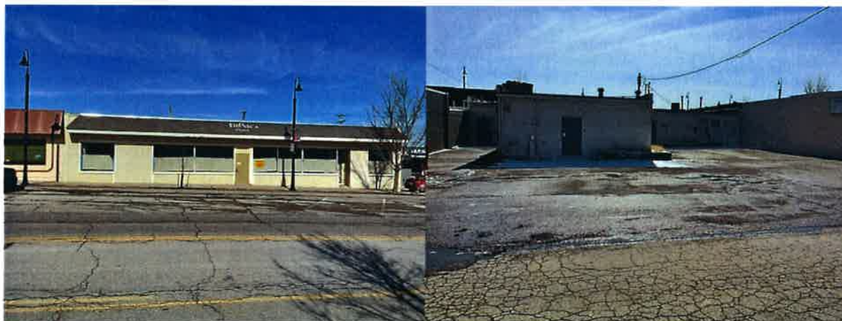
Figure 2 – Site Photos – (L) Storefront on 63 rd Street. (R) Rear of Property on Public Alley
